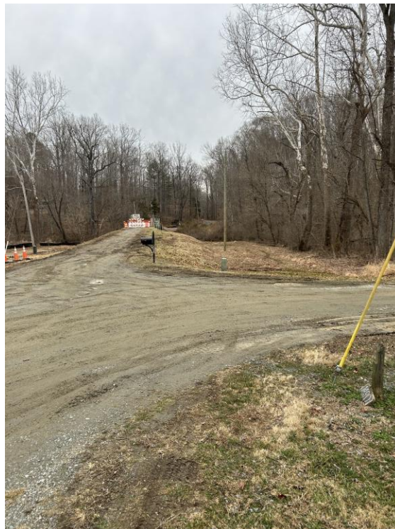
Figure 12. Vegetative clearing on Lecky Property (Hard Bargain), looking east
